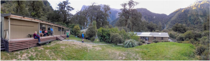
Dumpling Hut – dining hall at left, bunkroom at right. Photo Credit Spen Walker & Jane Bruce
